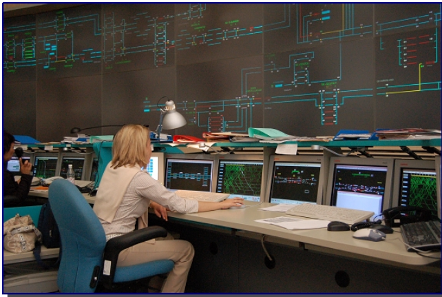
Figure 2. Operator and synoptic frame in Genoa's SCC.
